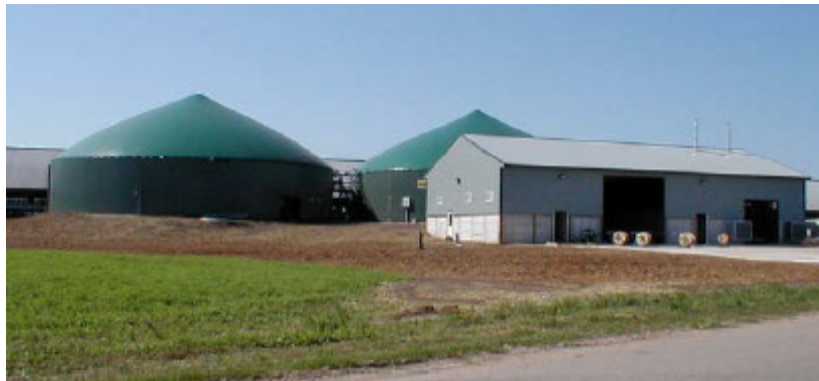
Scenic View Dairy, MI -Biomethane project
