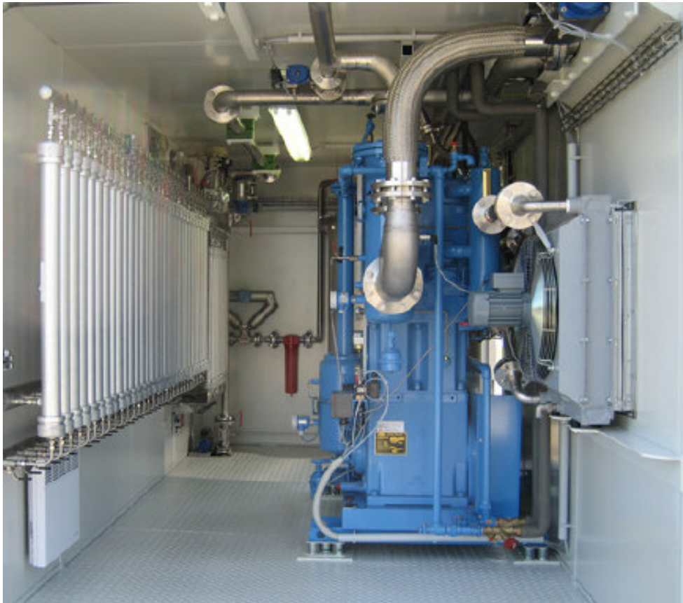
Figure 3. Demonstration plant for biogas upgrading with membrane technique. The plant was commissioned during fall 2007 in Bruck, Austria.
